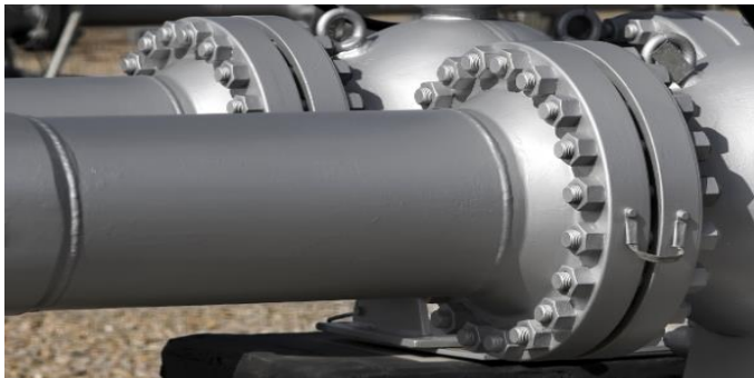
Figure 69. Application of studs
